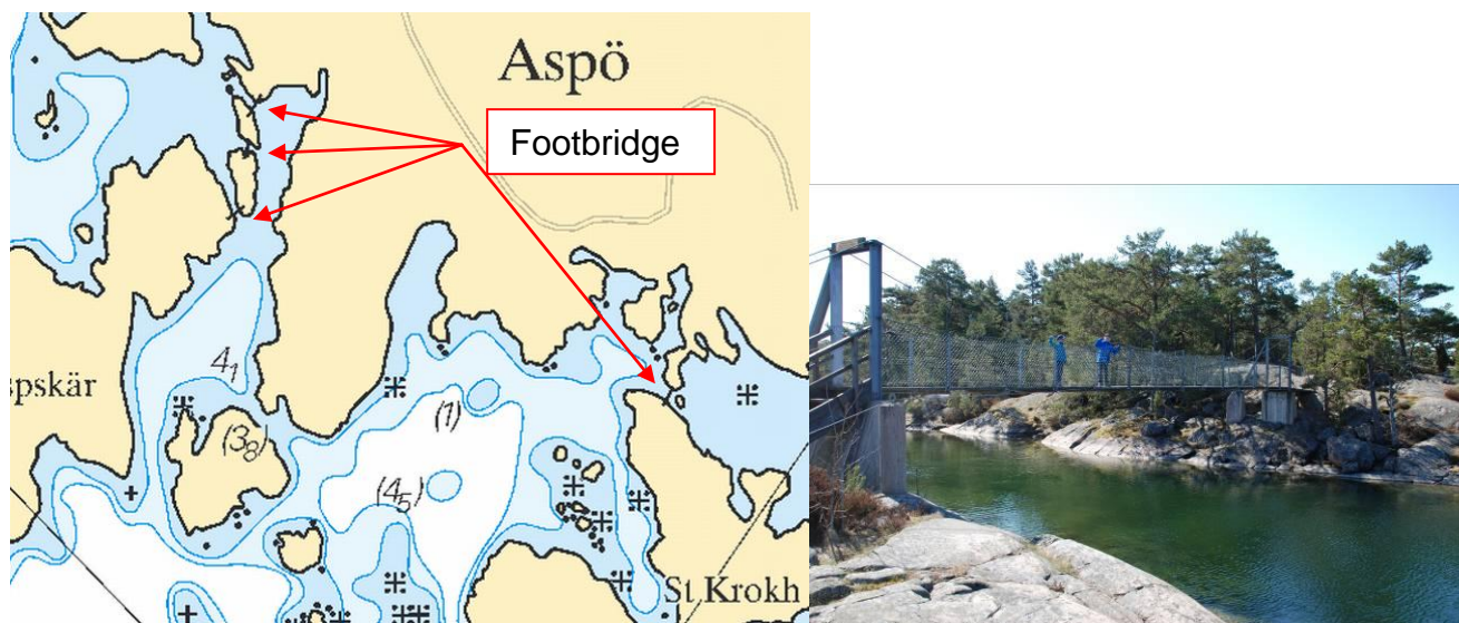
Image 1 Footbridge in a nature reserve in the Swedish archipelago
