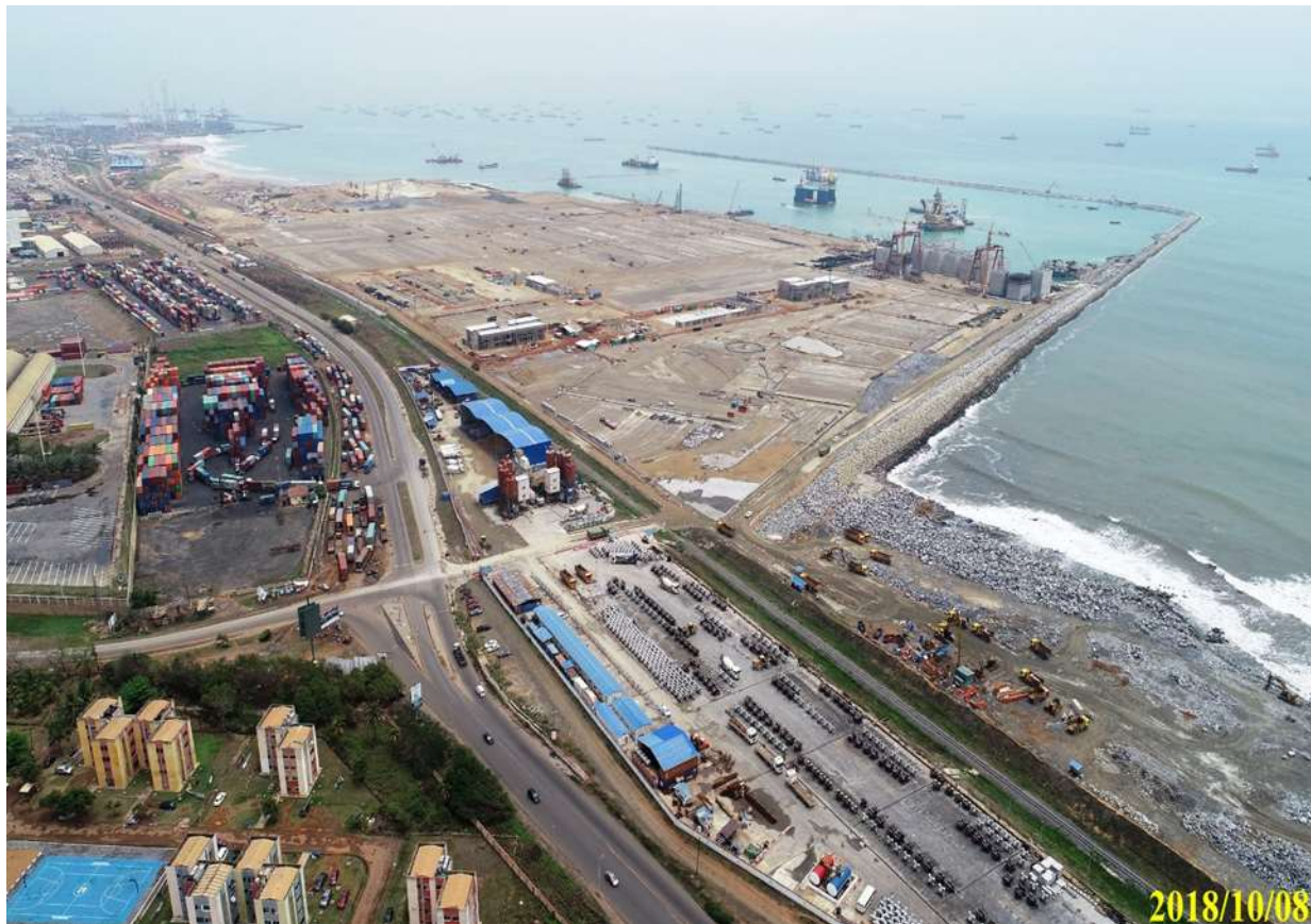
On –going Port Expansion project in Tema
