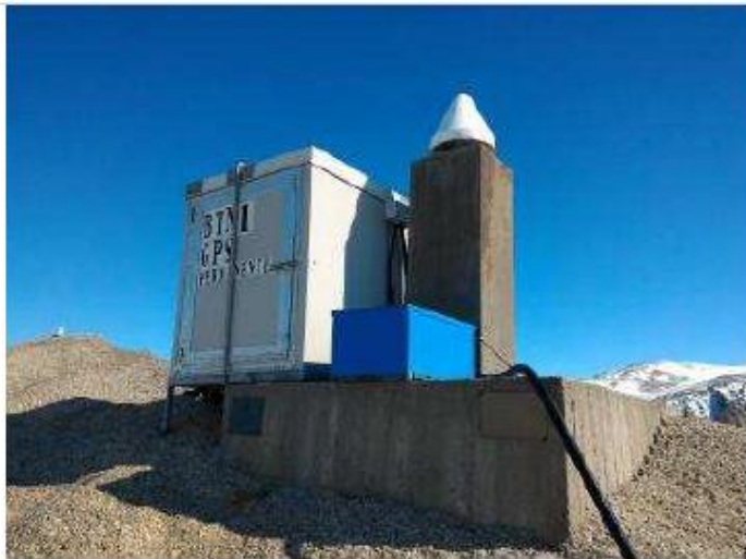
TNB1 continuous station monumentation
