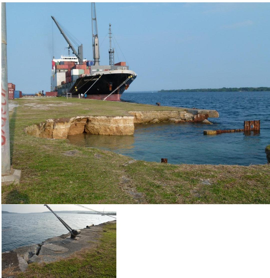
**Figure 7-1 : Mooring Bollards Need Upgrading at Main Wharf, Luganville for Large Vessels
