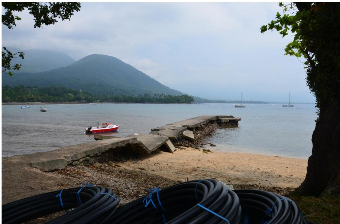
Figure 4-2 : Jetty at Sola, built in 1997. Undermined and Damaged by a Cyclone, 2011
