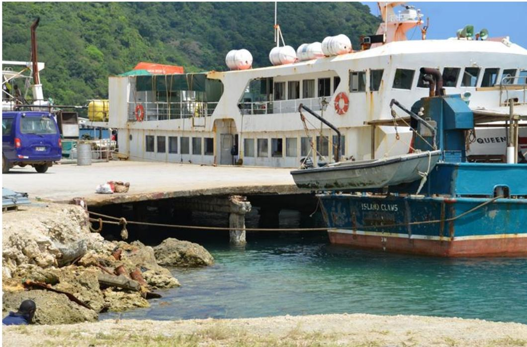
Figure 4-4 : Star Wharf is of Light Construction and in Poor Condition
